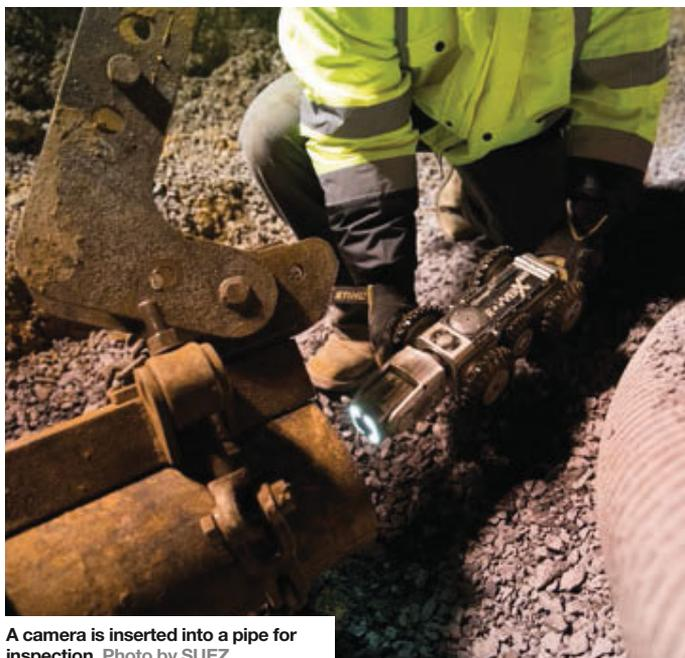
A camera is inserted into a pipe for inspection. Photo by SUEZ
