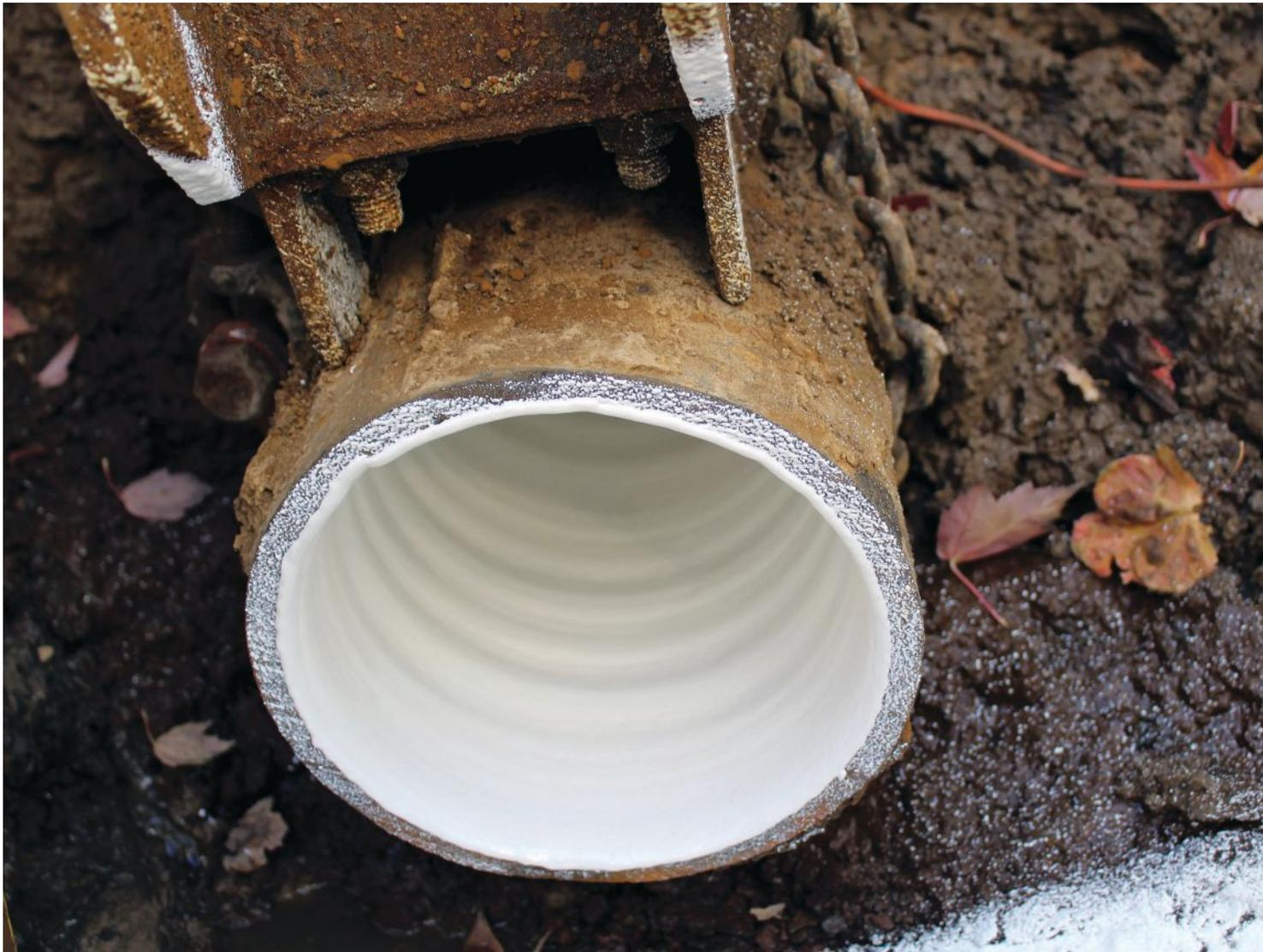
Once cured, this coating creates an internal seal that prevents leaks and helps protect against future corrosion and biological buildup. This extends the pipes' service life, helps reduce the frequency of maintenance, and increases the flow capacity for greater system efficiency.
