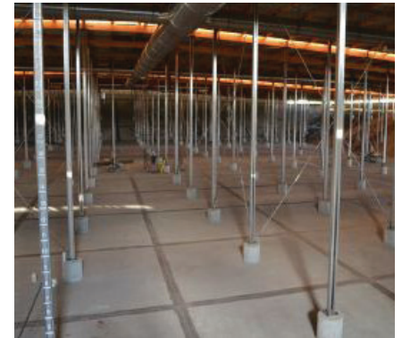
Empty More Ave. reservoir during installation of in-tank aeration systems.
