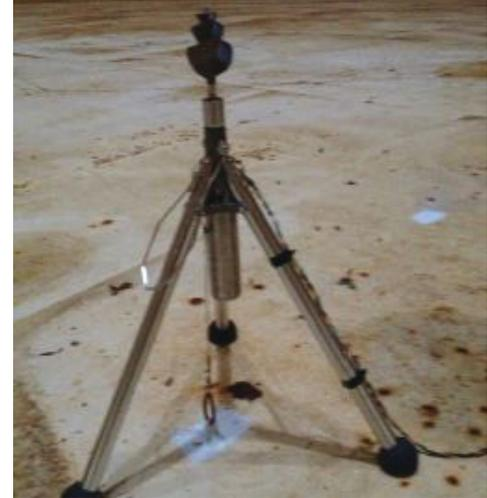
Figure 2a, b. Components of the TRS include a network of header pipes and spray nozzles installed on the roof of the tank and the PAX Water Mixer installed on the floor of the tank.
