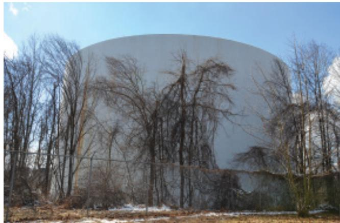
Figure 1. The 8 MG Hunting Hill tank has a high water volume and low turnover, which results in high water age and elevated THM levels
