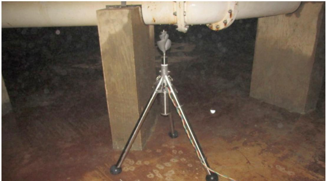
Figure 2. The PAX Water Mixer was installed in a 5MG tank with an existing passive mixer (shown behind PAX Water Mixer in above image).
